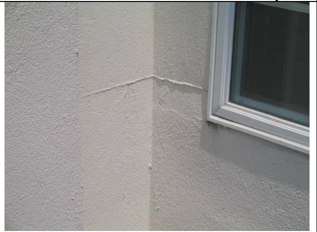
Photo 16. Stress Cracks
