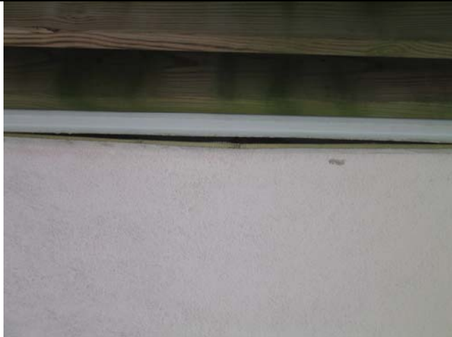
Photo 19. Sagging Soffit
