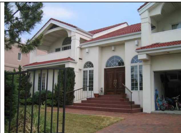
Photo 1. Front Left Corner
